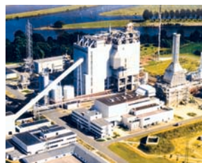
IGCC with Shell Coal Gasification.
